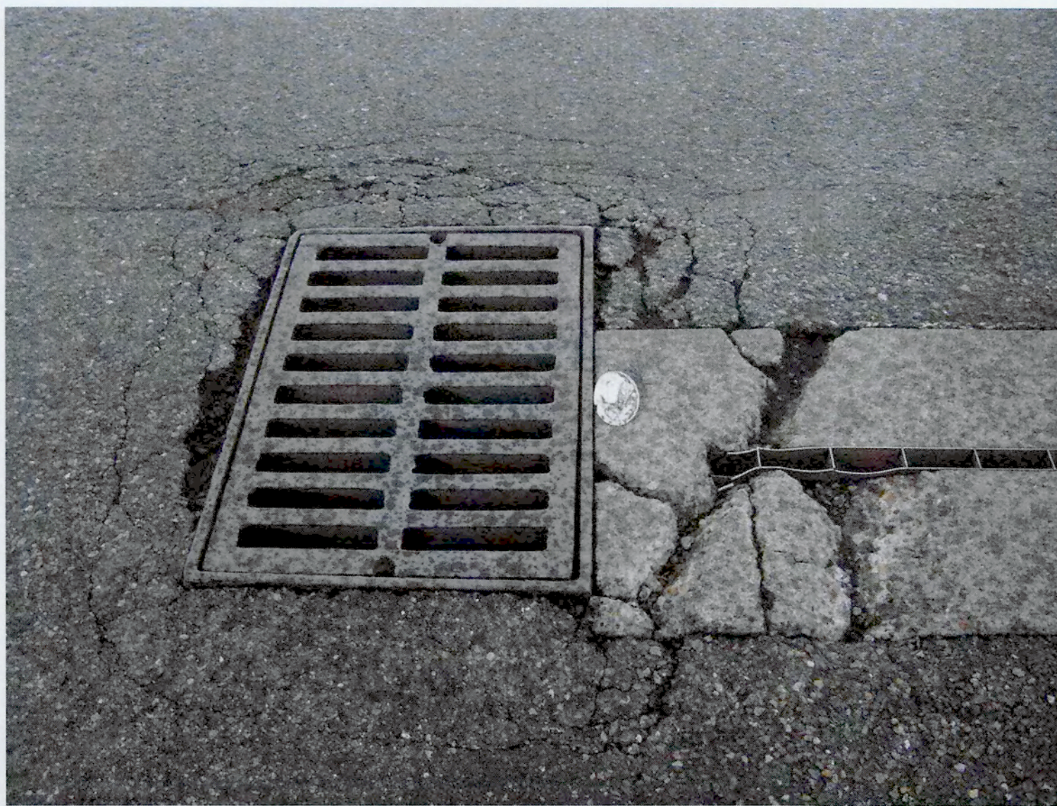
PHOTO - EXAMPLE EXISTING CONDITION
